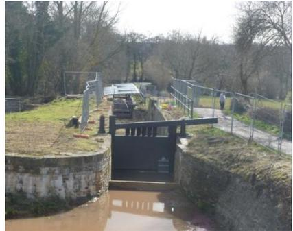
*Lower Brake Lock in the foreground with the top gate installed. Ty Coch Bottom Lock in the background with scaffolding and cover sheets in place (Pat Cleary)*
