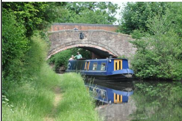
Gravelly Way Bridge on the Staffs & Worcs in the area affected by the proposed development
