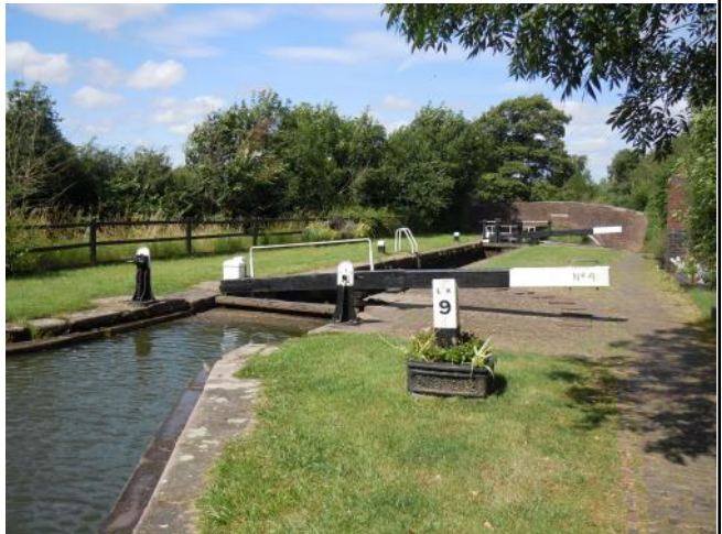
Curdworth Lock 9 and Cheatles Farm Bridge
