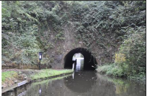
Curdworth Tunnel—East Portal
