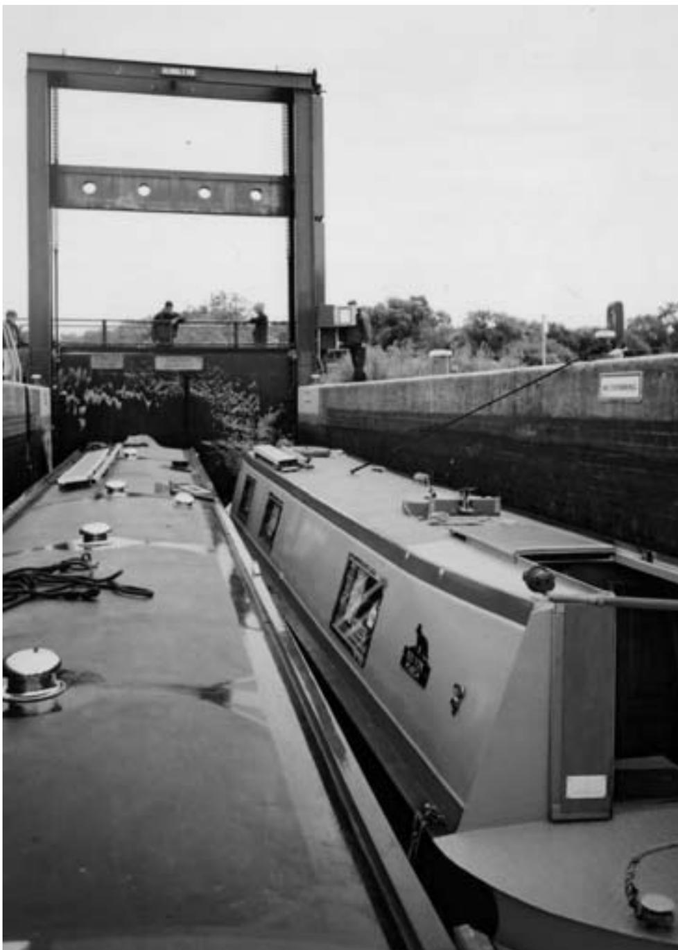
Instructions for lock operation are clearly displayed and straightforward. The lock must be left with the V gates upstream closed and the guillotine gates downstream fully open. If however on approaching the lock the V gates are chained back open and the guillotine gates partially lifted the lock has been 'reversed' and no attempt should be made to navigate. This is done in times of flood.
