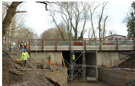
Photo: Working party volunteers set up scaffolding at Compasses Bridge ready for the bricklayers.
