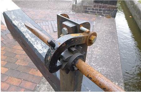
Photo: A pawl stop fitted to the paddle gear at Planet Lock on the Caldon Canal in Stoke-on-Trent
