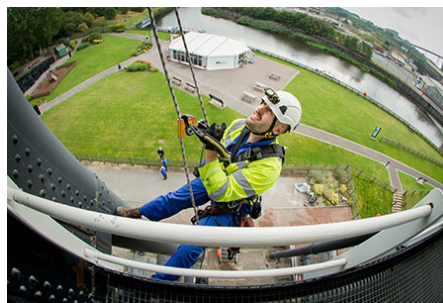
Photo: Abseilers Inspect the Anderton Boat Lift
