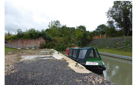
Photo: The Blocked Section of the Canal Basin at Nelson's Wharf on the Grand Union Canal at Stockton
