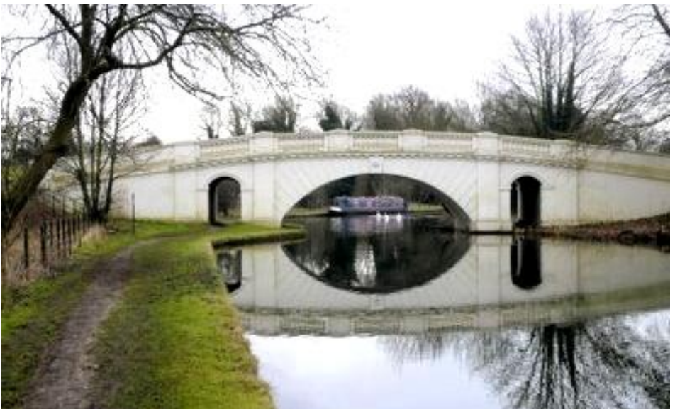
The elegant curves of The Grove Bridge on the Grand Union near Watford.
