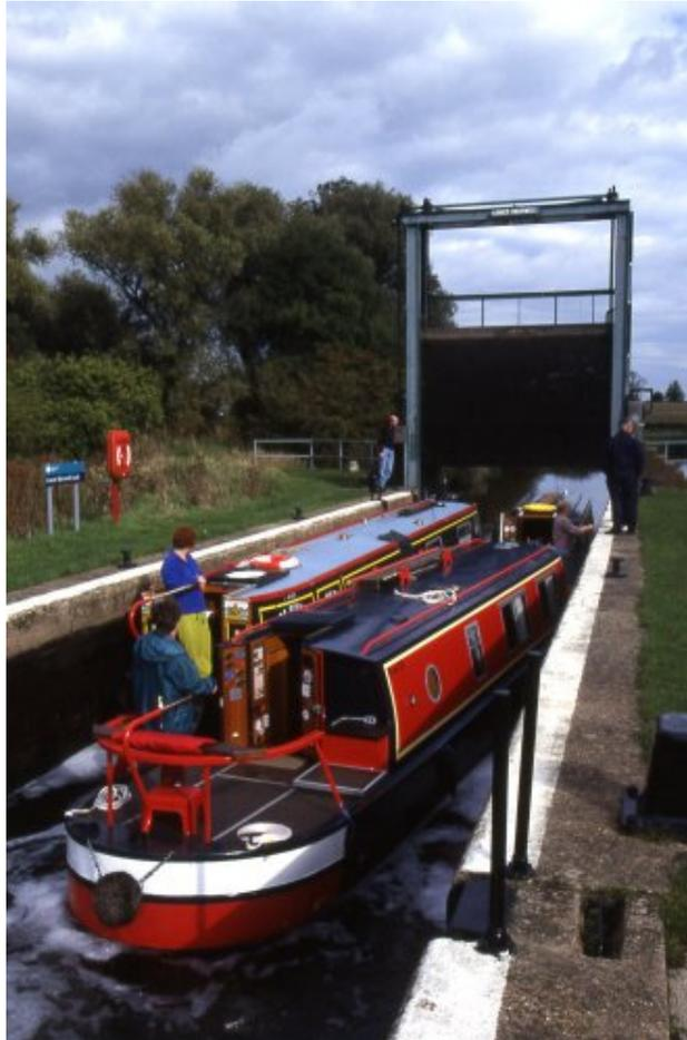
**Lock Sizes and maximum craft dimensions:** Length 78 foot, beam 14 foot. Note - Irthlingborough Bridge restricts the maximum beam of craft navigating the Nene to 13 foot.
