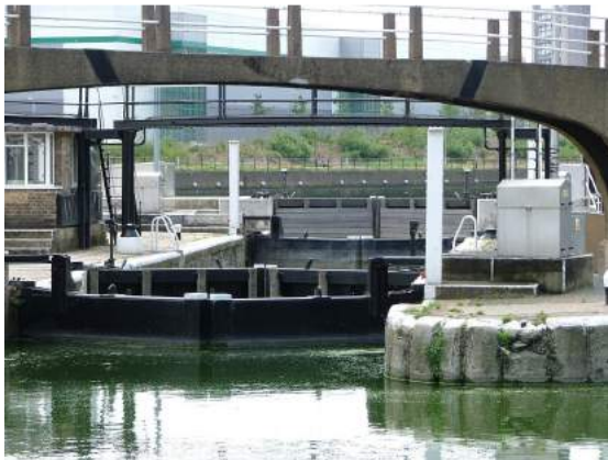
New outer gates fitted at Bow Locks were designed to protect the Lee Navigation and surrounding land from predicted higher tidal surge levels in the future
