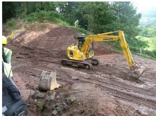
Embankment failures on canals present risks to life and property and repairs are often costly, as seen on the Monmouthshire and Brecon Canal in 2008
