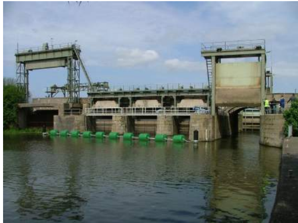
Some infrastructure serves both navigation and water management functions, as here at Denver Sluice, where management of flows is crucial to limitation of sedimentation in the tidal Great Ouse navigation downstream, as well as for flood management and maintenance of public water supplies
