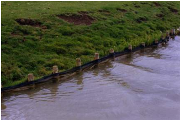
Geotextile bank protection limits erosion by boat wash, while reed planting behind can create a buffer for land run-off
