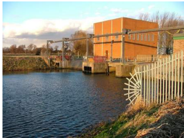
Many fenland waterways are also key 'high level carriers' conveying water pumped from adjacent lower-lying land
