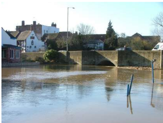
Almost complete loss of headroom at historic bridges during floods, as seen here on the Warwickshire Avon at Tewkesbury, inevitably causes closure to navigation
