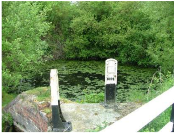
Restoration and use of historic side ponds at locks could save water. This principle is also used in 'economiser' locks on major modern waterways in continental Europe.
