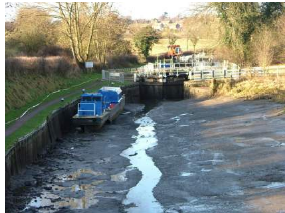
Lock gate replacement at Braunston – prevention of leakage at locks will become increasingly important
