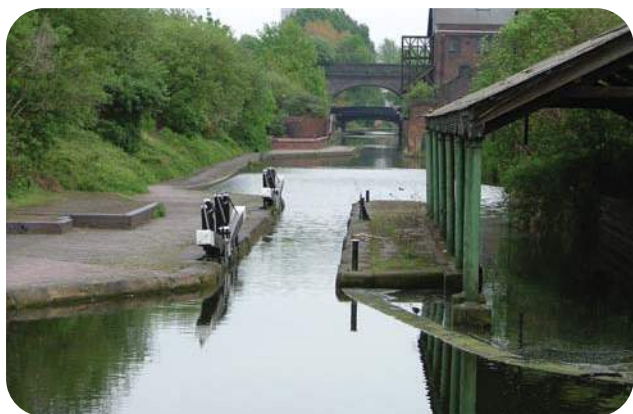
Urban waterways often have highly reinforced banks and some are impacted by a cocktail of pollutants. Both reduce their ability to support rich wildlife communities
