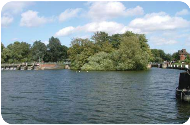
Weirs and locks were built on rivers such as the Thames to improve navigation
