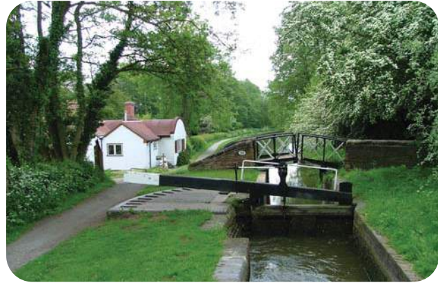
Many waterway structures are listed, including this cottage and split lock bridge on the Stratford Canal
