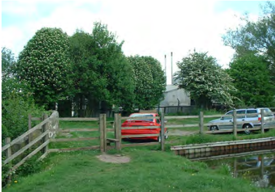
Current terminus of Leek Arm at Barnfields Aqueduct.
