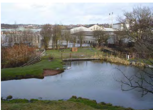
View from canal feeder towards aqueduct and existing canal terminus
