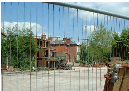
Former Churnet Valley Public House. Viewed across IAE's yard.
