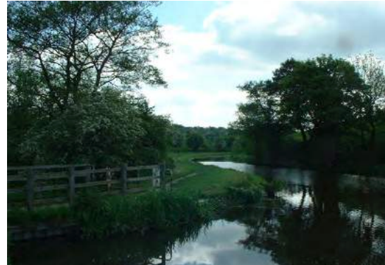
View east along canal from aqueduct.
