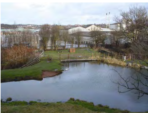
Existing terminus of Leek Arm at aqueduct.
