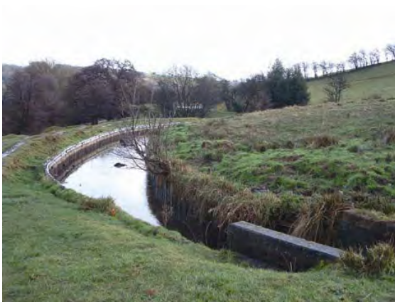
Canal feeder and culvert
