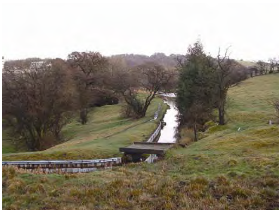
View east along canal feeder towards aqueduct
