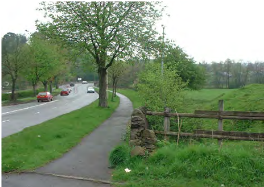
A53 towards Leek town centre. Area for proposed basin is located to right.
