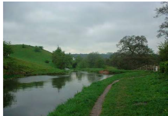
View west along canal to Barnfields Aqueduct and feeder.
