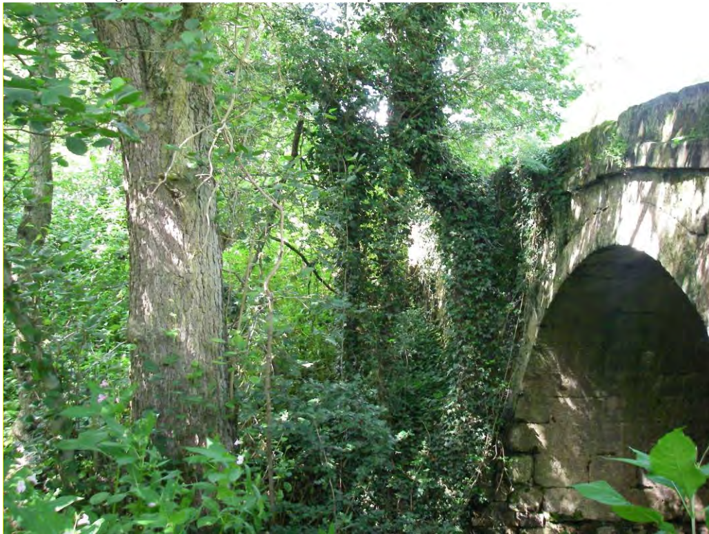
Plate B.1: Bridge arch and elevations sheltered by trees
