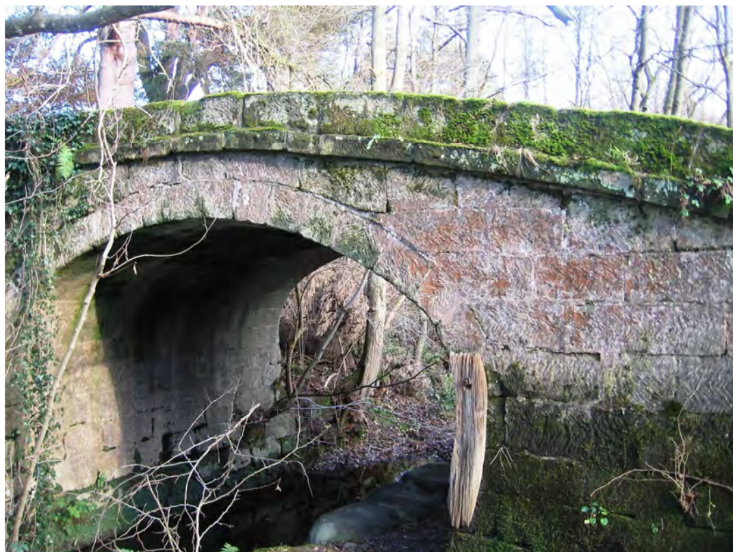
Photo(20): West elevation, south spandrel in good order.
