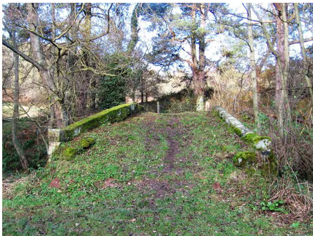
Photo(2): Bridge Deck from South approach
