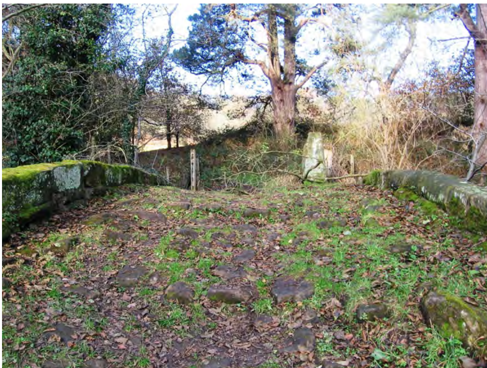
Photo(3): Bridge Deck surfacing clay and large stone undressed blocks.
