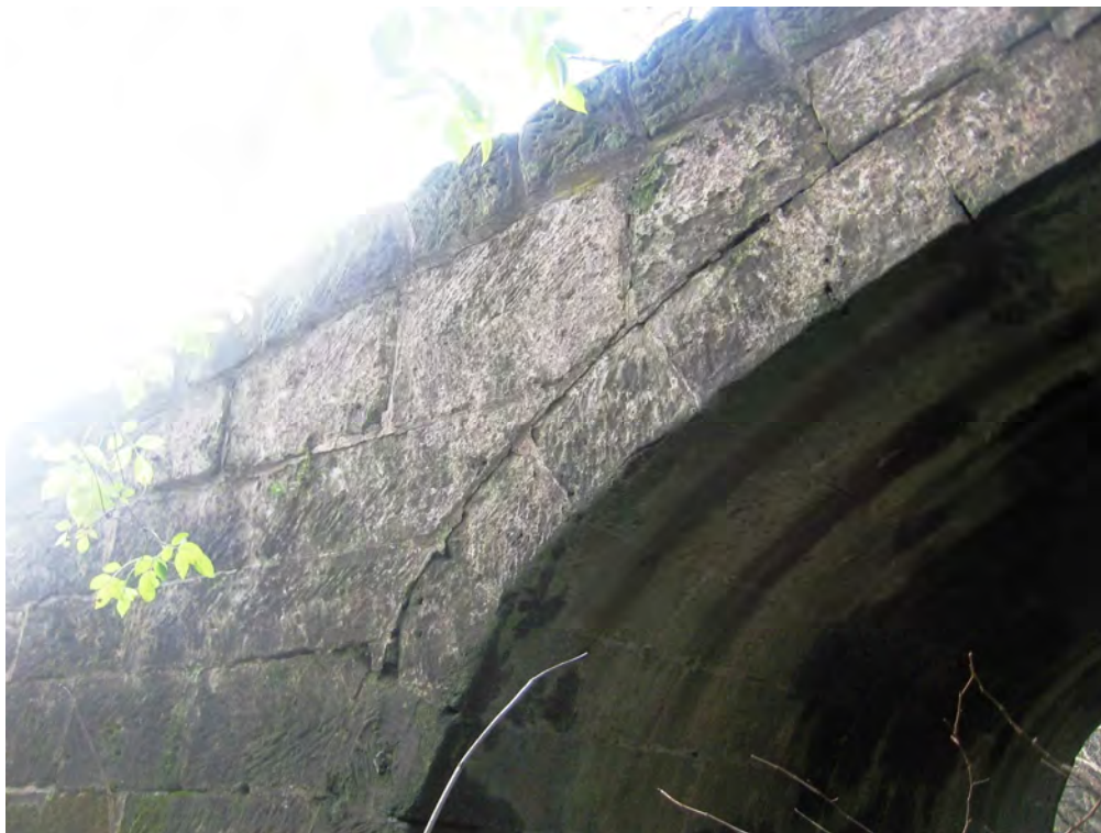
Photo(11): East elevation, south spandrel in good order.
