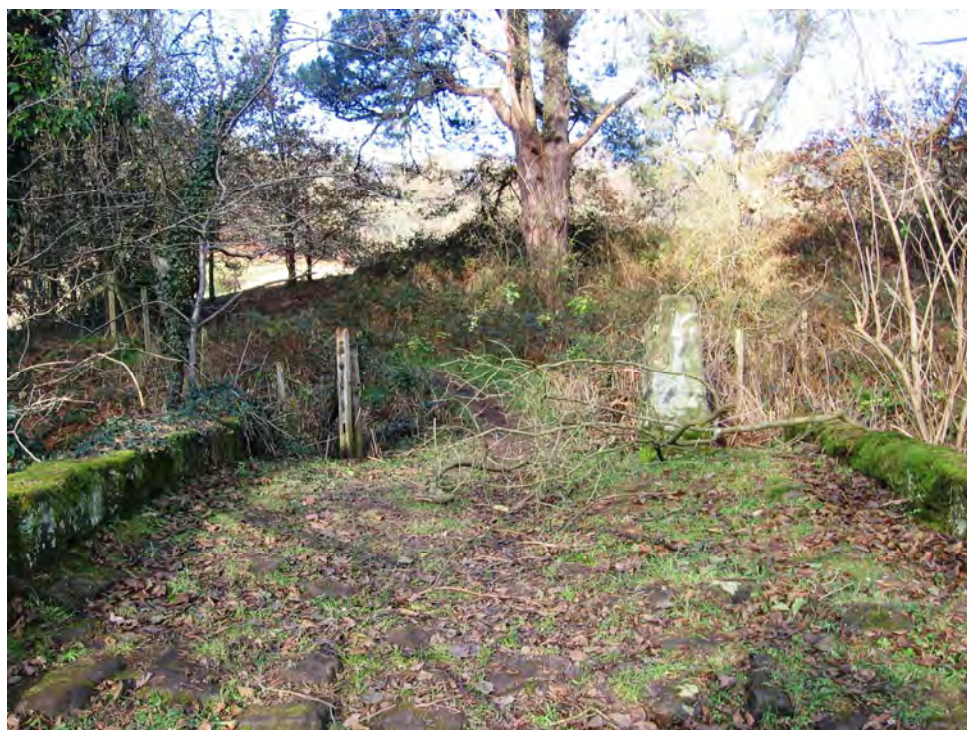
Photo(4): North approach viewed from bridge deck.
