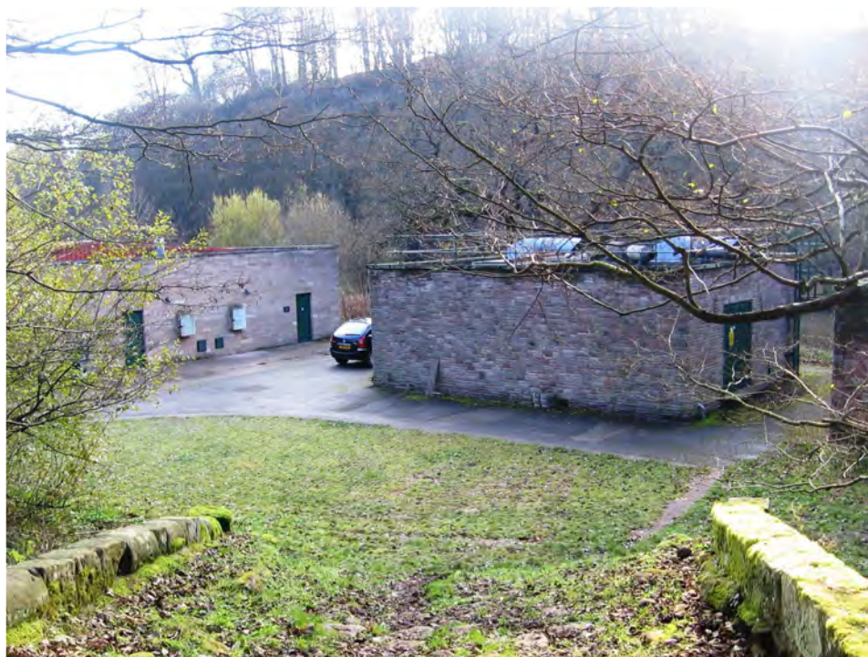
Photo(6): South approach and pumping station from bridge.
