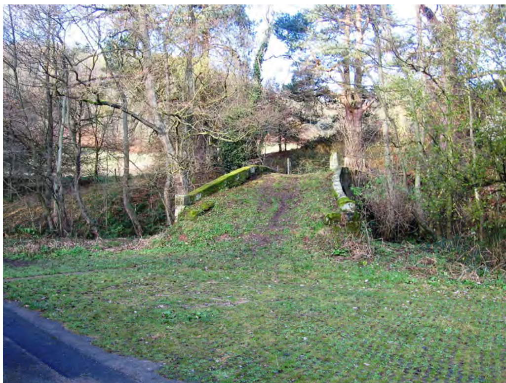
Photo(1): Bridge Deck from Pumping Station.
