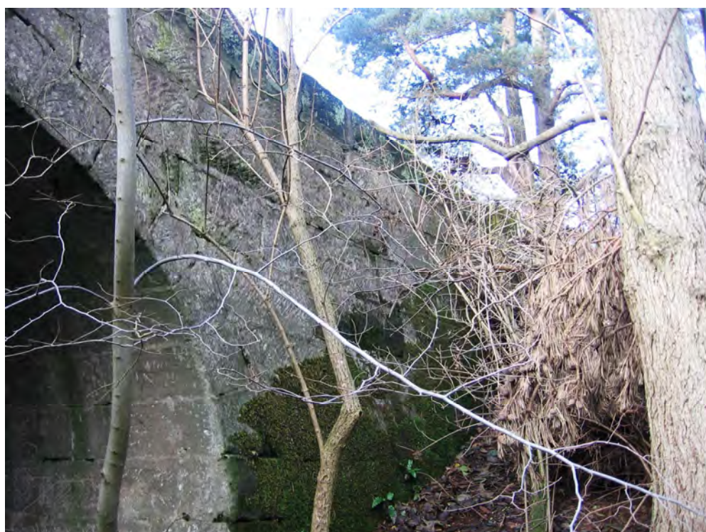
Photo(12): East elevation, north spandrel in good order.
