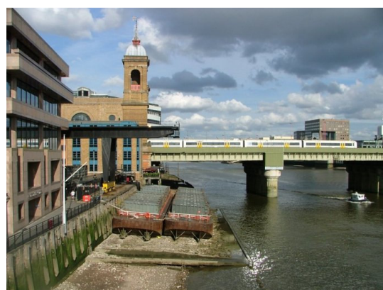
This refuse wharf in the City of London loads barges with containers across the Thames Path. However, the path is maintained with a protected passage (just visible) and traffic lights/barriers for occasional brief closures
