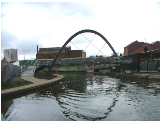
Surfaced towpath and new bridge over the canal in Coventry suitable for use by both cyclists and walkers
