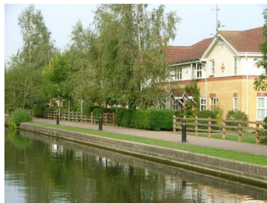
Modern development on the non-towpath side of the Grand Junction Canal incorporates a waterway path accessible to all, although this is not a PROW
