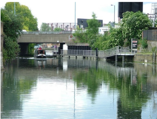
The need to cross a busy road on the level where there is no towpath under the bridge has been overcome here on Limehouse Cut in London by use of a floating path
