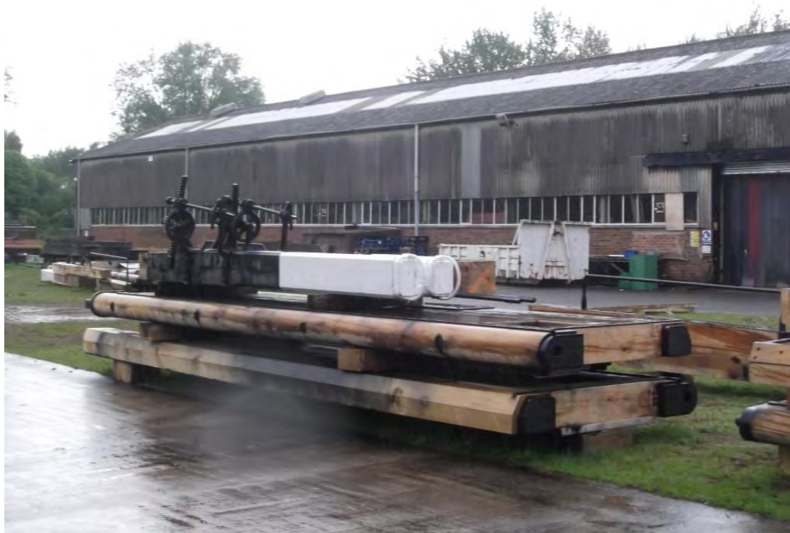
Figure 5: New lock gates at Bradley Yard
