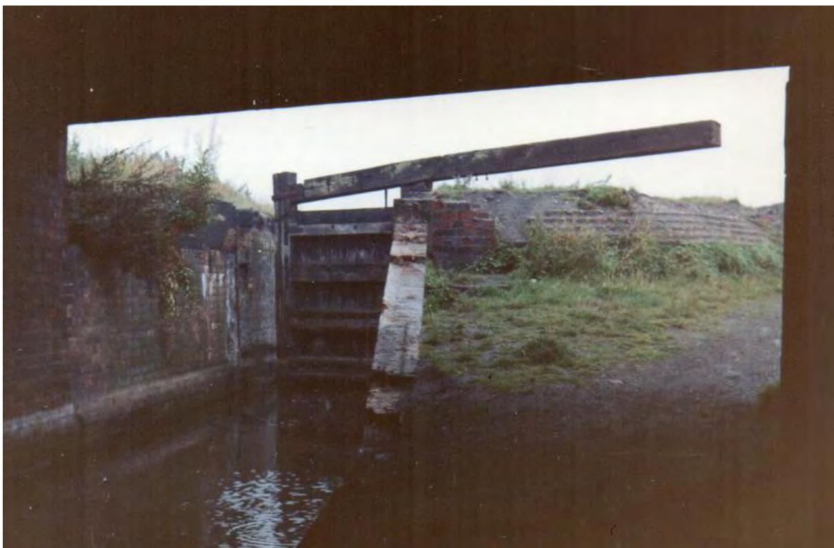
Figure 4: Bradley Lock 7 and Great Bridge Crossing circa 1960
