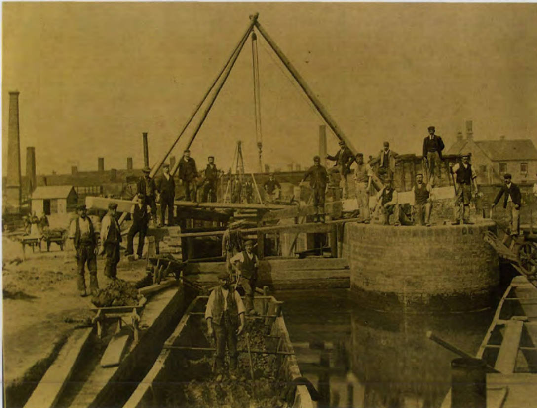
Barge Lock reconstruction to the lock approaches in 1905 © Worcester Record Office
