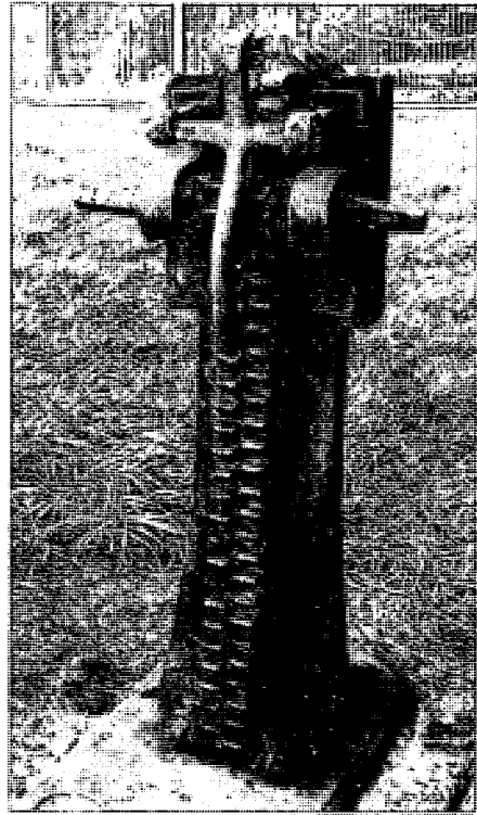
Square ended alternative stand at Diglis Basin Barge Lock with original components © David McDougall
