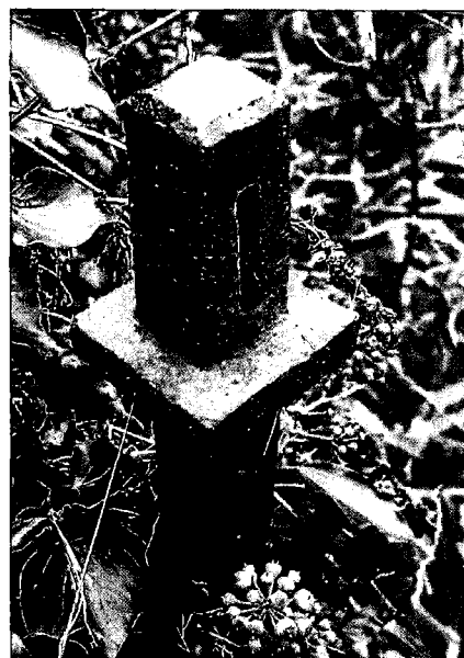
Paddle rod termination at Mildenhall Mill © David McDougall
