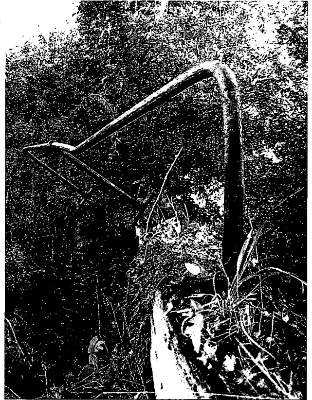
Lock 7 surveyed handrail on top gate
