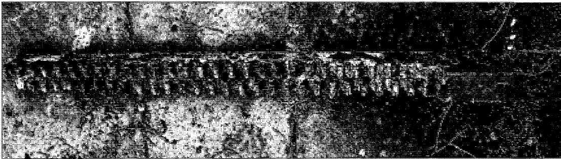
Broken rack of Worcester & Birmingham Canal origin © David McDougall
