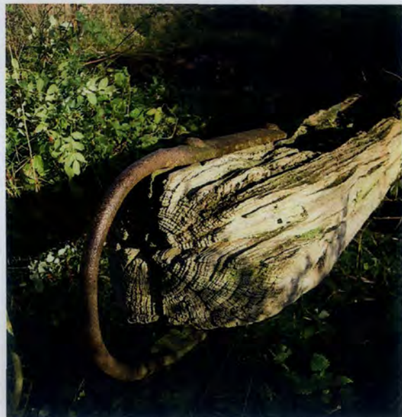
Top gate balance beam at Lock 7 has a curve offsetting the beam by 12 inches (300mm) at the end. The handhold is forged from D section wrought iron and riveted through the beam depth.
