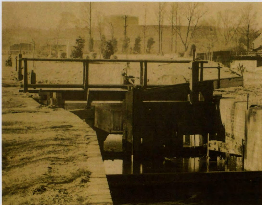
Enlargement of 1939 view of derelict Barge Lock to show paddle gear © Worcester Record Office
