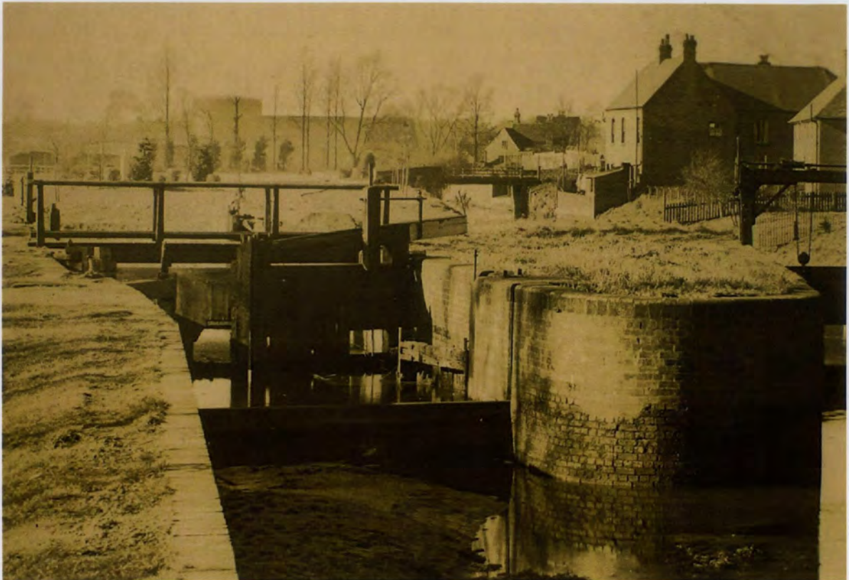
Decayed gates at the Salwarpe end of the Junction Lock in 1939 © Worcester Record Office
