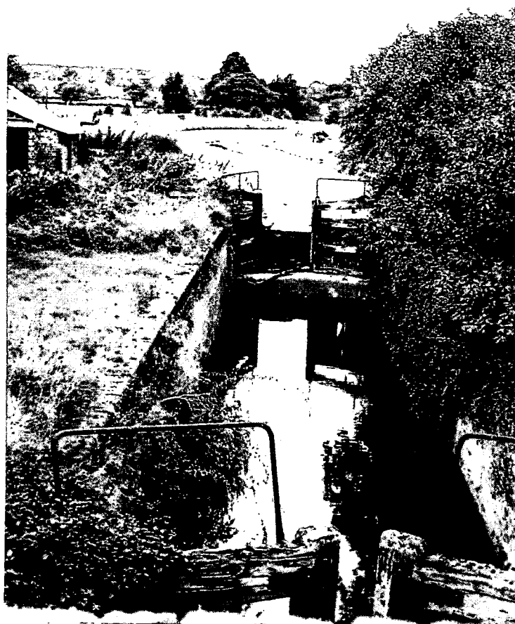
Porter's Mill Lock No 5 1956 Three bar top gates
