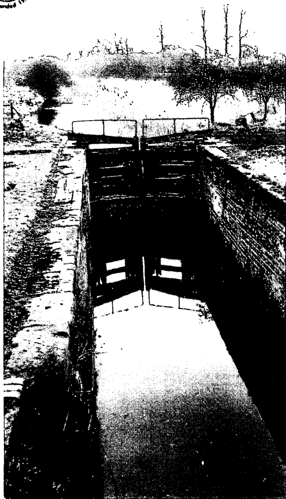
Ladywood Top Lock No 1 1947 Four bar top gates
