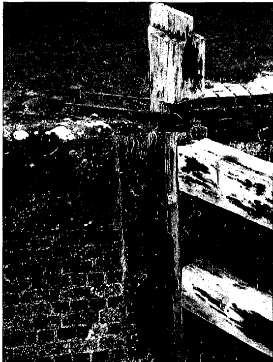
Collar forging at Mildenhall Mill Lock 6 retaining replacement top gate. Note cast iron quoin. © David McDougall
