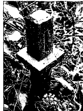
Rack fitted to end of gate paddle bar with cotters bent over to secure them.
