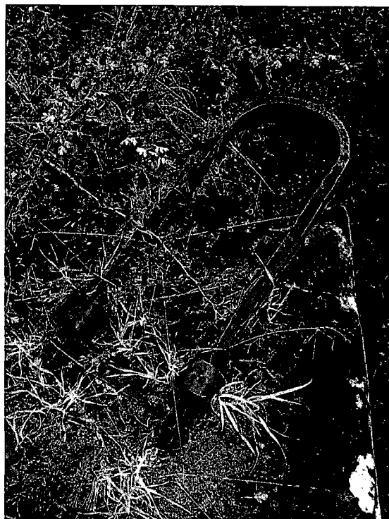
Collar forging in situ at Hawford Lock 7. Two of the staples have sheared off. © David McDougall
