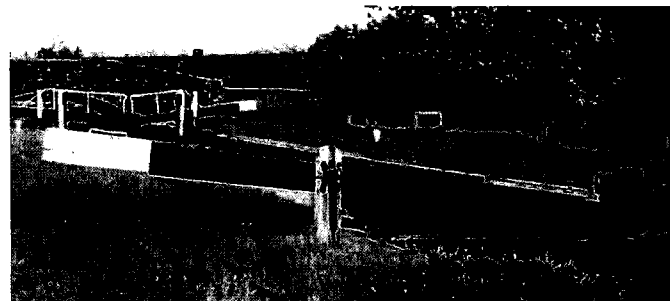
Top: Staffs & Worcs Canal wooden ground paddle jackheads 1977 Swindon Lock © David McDougall Bottom: Whitsunday Pye Lock 1970 Arthur Watts Collection © Waterways Archive Gloucester
