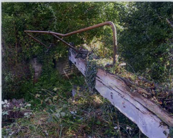
Top gate balance beam at Lock 7 has a curve offsetting the beam by 12 inches (300mm) at the end. The handhold is forged from D section wrought iron and riveted through the beam depth.
