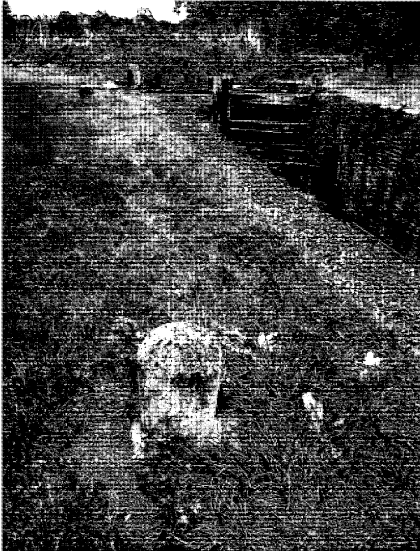
Concrete bollards at Mildenhall Mill Lock © David McDougall 2007
