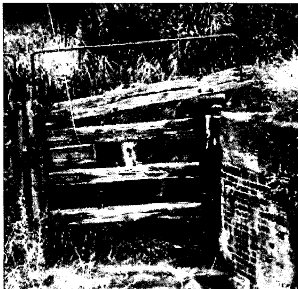
Derelict gate Lock 1 at Ladywood showing iron straps and 'L' plates in lower corners © RM Sinclair
