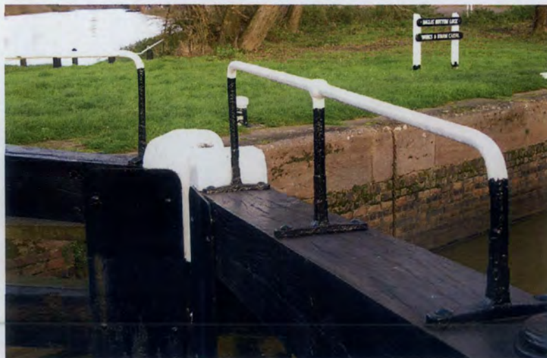
Diglis Locks, Worcester. Worcester & Birmingham made handrail in wrought iron © David McDougall
