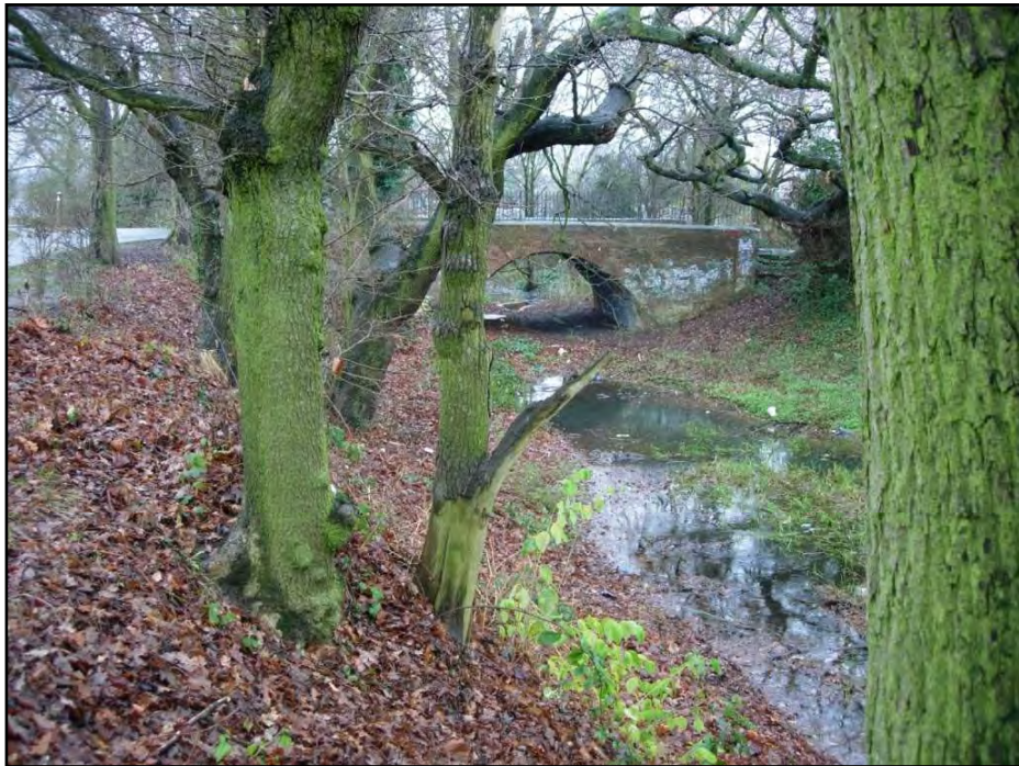
Figure 2.4 – Selly Park Bridge from south side of proposed Harborne Wharf
